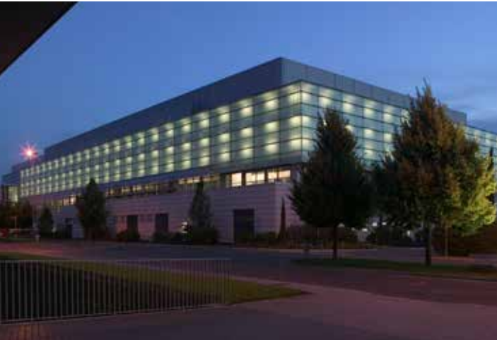
FERRARI PAINTSHOP BUILDING - MARANELLO (MO)
